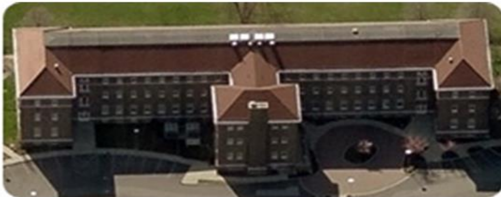
Figure 4-5. Building 101 in the Navy Yard in Philadelphia (EEB Hub, 2013). All rights reserved. Reproduced here for educational purposes only.
